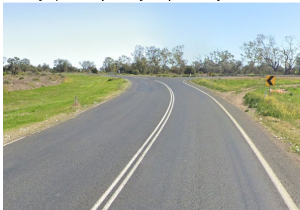
Photograph 1: Gwydir Highway Looking West
